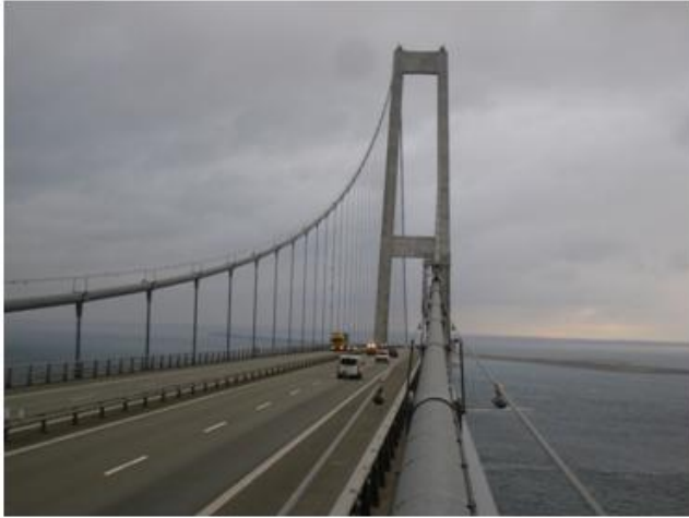
Structural Fatigue Monitoring
